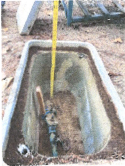
6 The correct way to set a backflow.jpeg 209K
