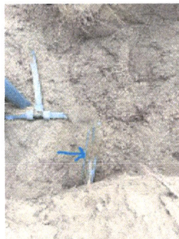
5 Tracer wire only on old line.jpeg 128K
