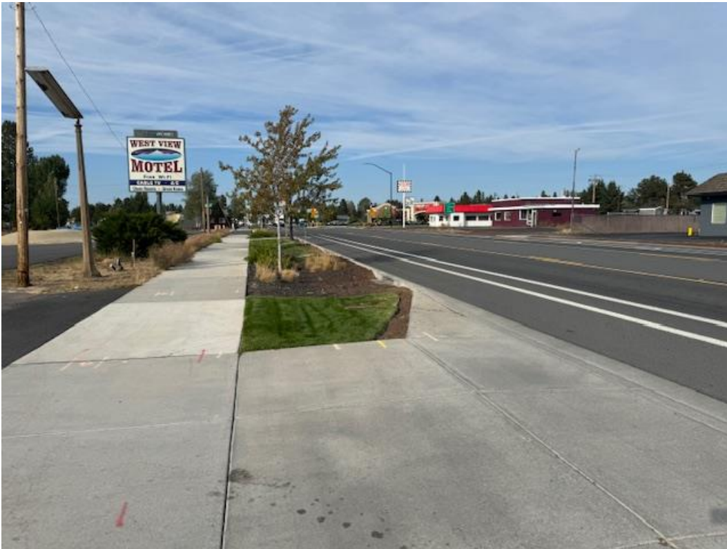
Figure 10. View from the shared US 97 access facing north.
