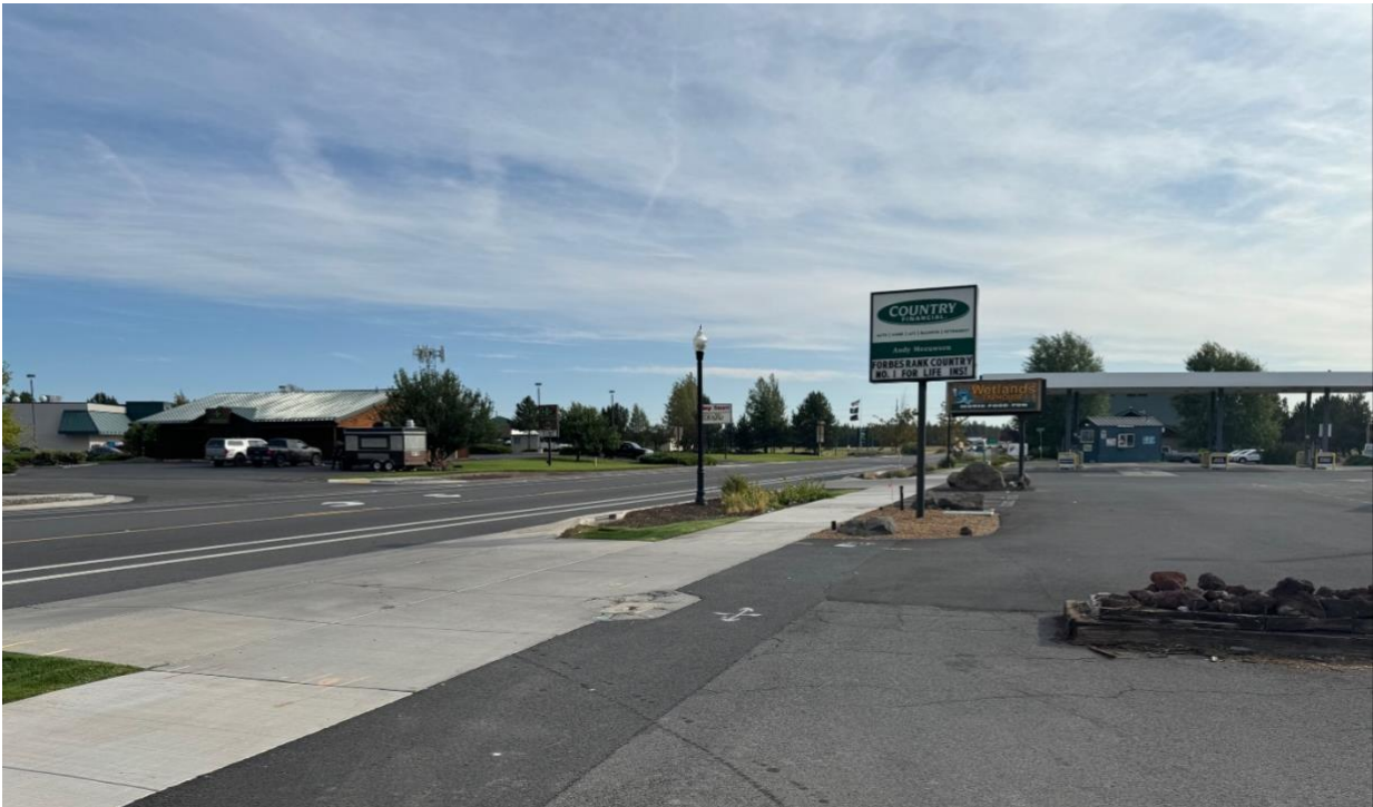
Figure 15. Existing internal splitter island near the shared US 97 access.
