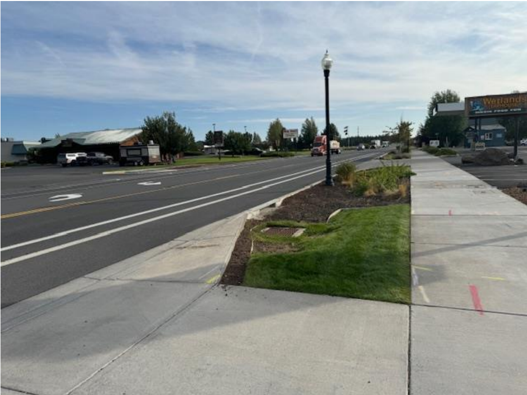
Figure 9. View from the shared US 97 access facing south.
