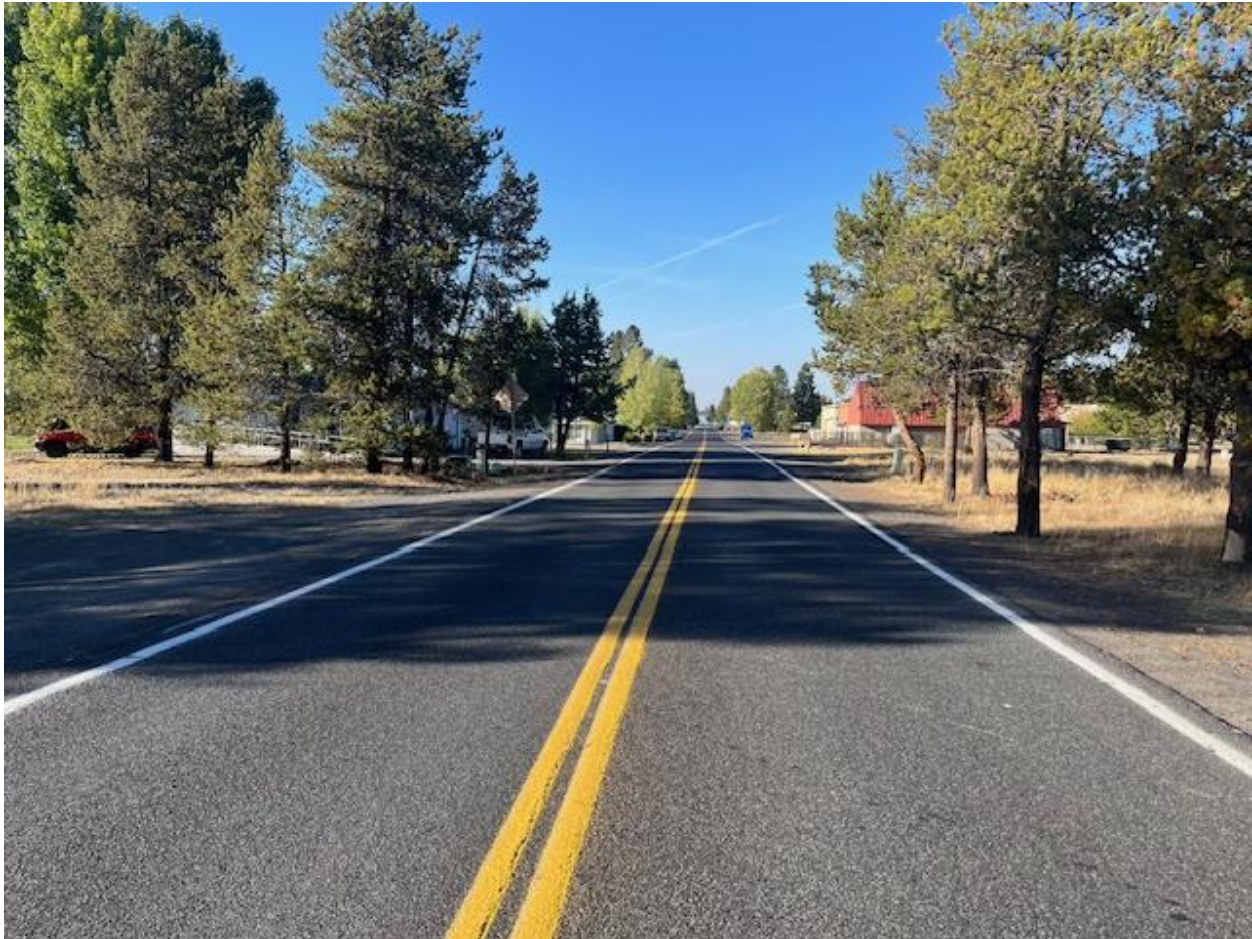
Figure 4. Morson Street streetscape north of the project site (facing north)
