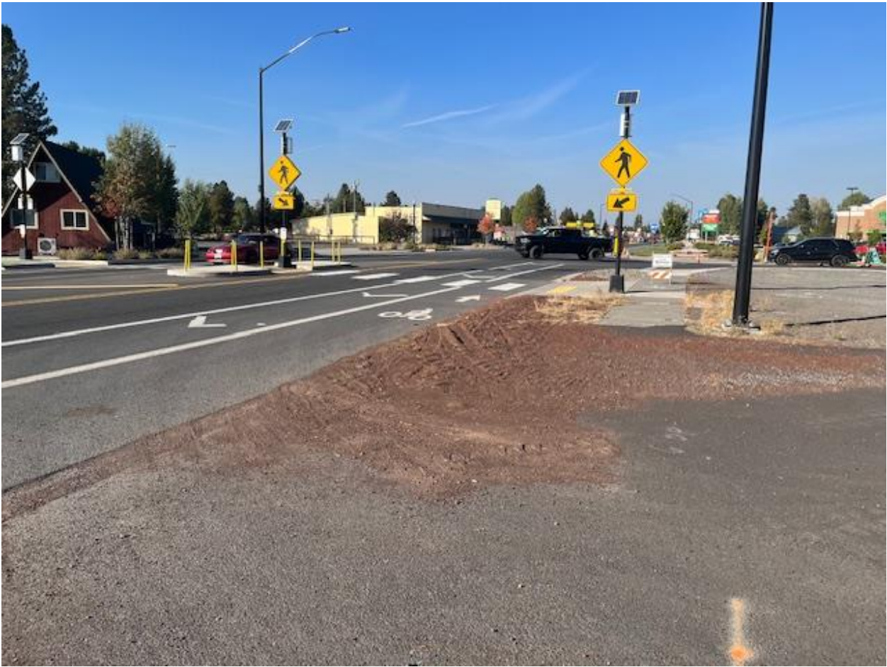
Figure 12. US 97/Finley Butte Road intersection facing south showing the recently installed raised pedestrian refuge island and sidewalks.
