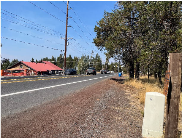
Looking North – Creeping Forward Beyond Utility Box
